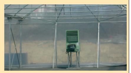
sary heating power has been obtained to achieve the desired thermal increase. In this way they can calculate the number of generators and the position in which to place them. The fuel for the installed generators is gasoil and has been approved and certified by the territorial industrial delegation.
